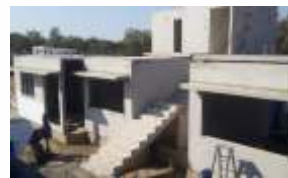
YOUR HOUSE INSTALLED ON YOUR SITE
